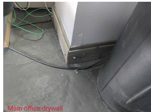
6. Main office drywall
