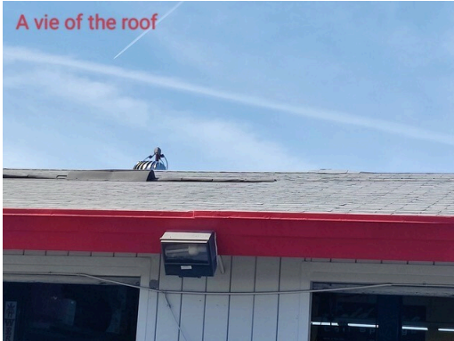
1. View of the roof
