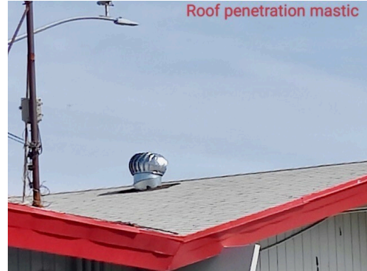
2. Roof penetration mastic
