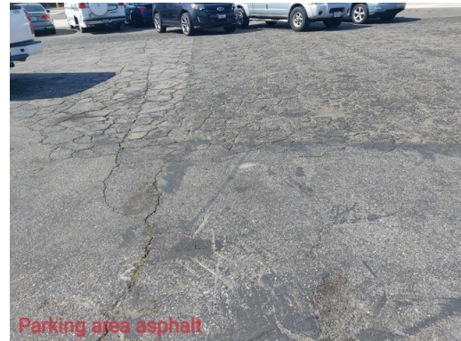
4. Parking area asphalt
