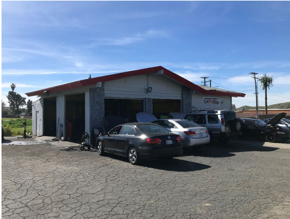
Photograph 1. Subject Property building.
