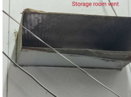
8. Storage room vent
