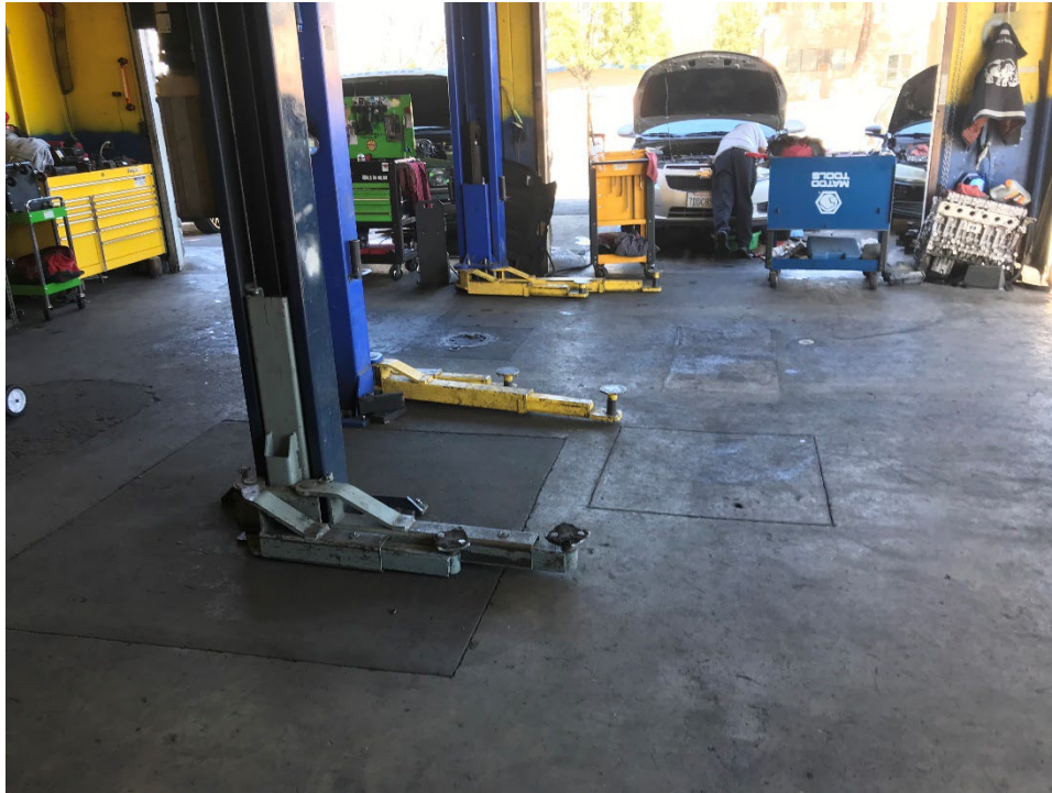
Photograph 13. Aboveground hydraulic lifts in the auto repair shop of the Subject Property building.
