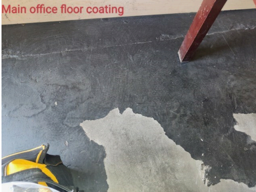
7. Main office floor coating
