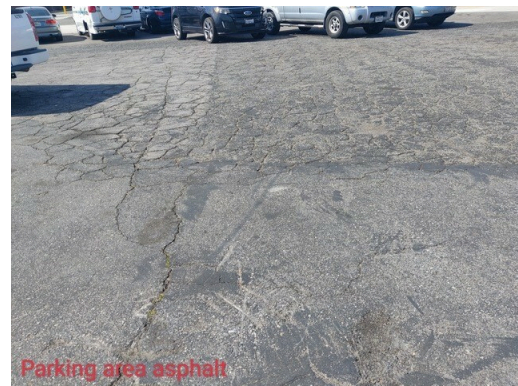
4. Parking area asphalt
