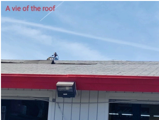
1. View of the roof
