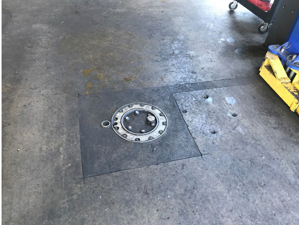
Photograph 15. Former in-ground piston lift in the auto repair shop of the Subject Property building.
