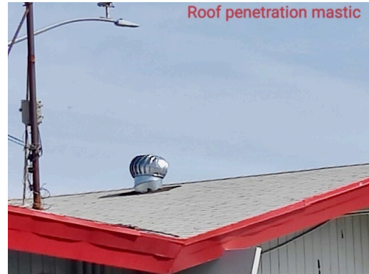
2. Roof penetration mastic
