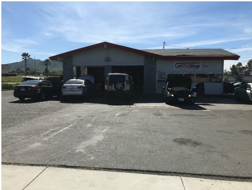
Photograph 2. Subject Property building, looking south.
