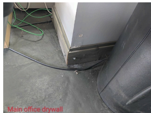
6. Main office drywall
